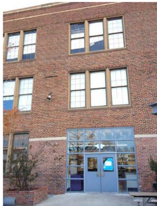
Original windows have been removed and new exterior doors and storefront installed in their place at west facade
