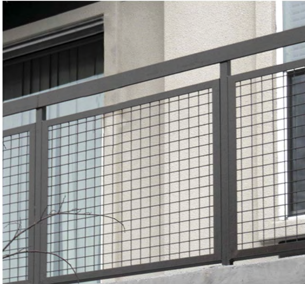
Balcony Handrails (Painted Steel—Warm Gray)
