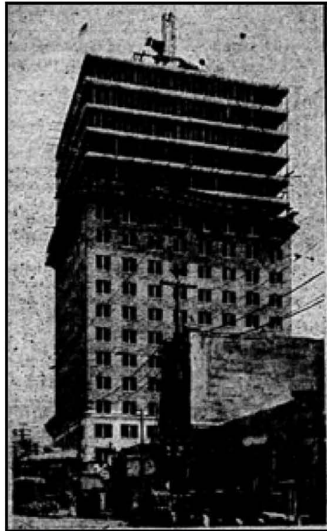
Figure 11. The Allen Building with brickwork completed to the fourteenth floor ( Dallas Morning News , 7 March 1926:1).
