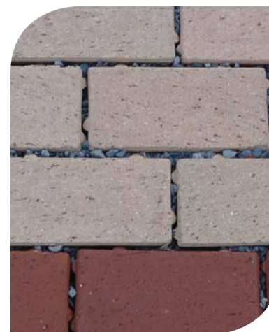
Pedestrian crosswalk with special pavers
