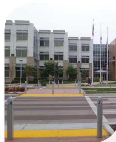
Pedestrian crosswalk with special pavers
