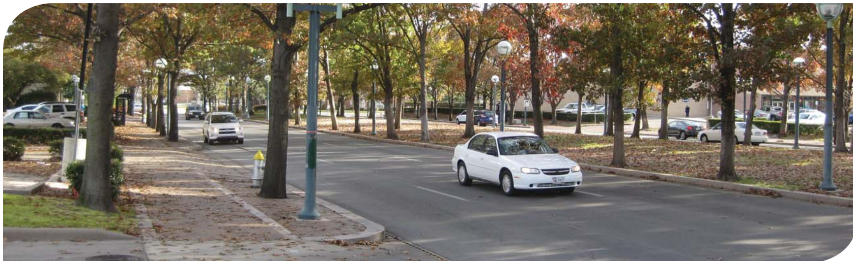
North Haskell Avenue at Capitol Avenue—six-lane divided thoroughfare with planting zone and sidewalks in a shopping strip environment
