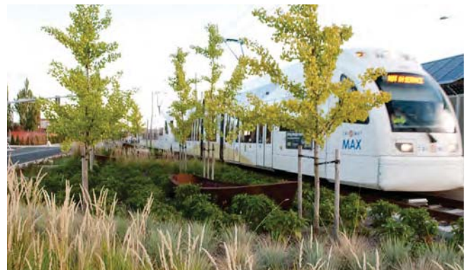
Light rail in Portland is built with iSWM adjacent to many of their tracks
