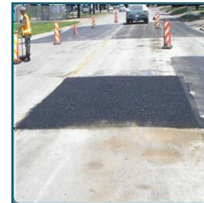
Full-Depth Asphalt Repair for "C" rated streets
