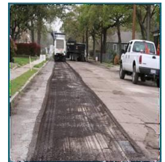
Asphalt Rehabilitation for "D" rated streets
