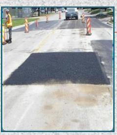
**Slurry Seal** - This treatment for CONCRETE STREETS WITH ASPHALT SURFACE consists of a ¼-inch layer of sand and fine stone mixed with asphalt emulsion. This seals and smooths the surface and conceals scars from previous repairs. It is used predominately for residential roads with curb and gutter. The work is outsourced to a specialized contractor – after Street Services performs preparation work (such as minor base repair and crack sealing).
