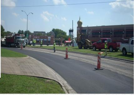
**Re-Surfacing** – This treatment removes the entire asphalt surface, and pulverizes and recycles the old material with new asphalt binder. The new asphalt surface is then placed over the entire surface, compacted, and smoothed to a proper finish. Curb and gutter repair, if needed, is accomplished with the re-surfacing efforts.
