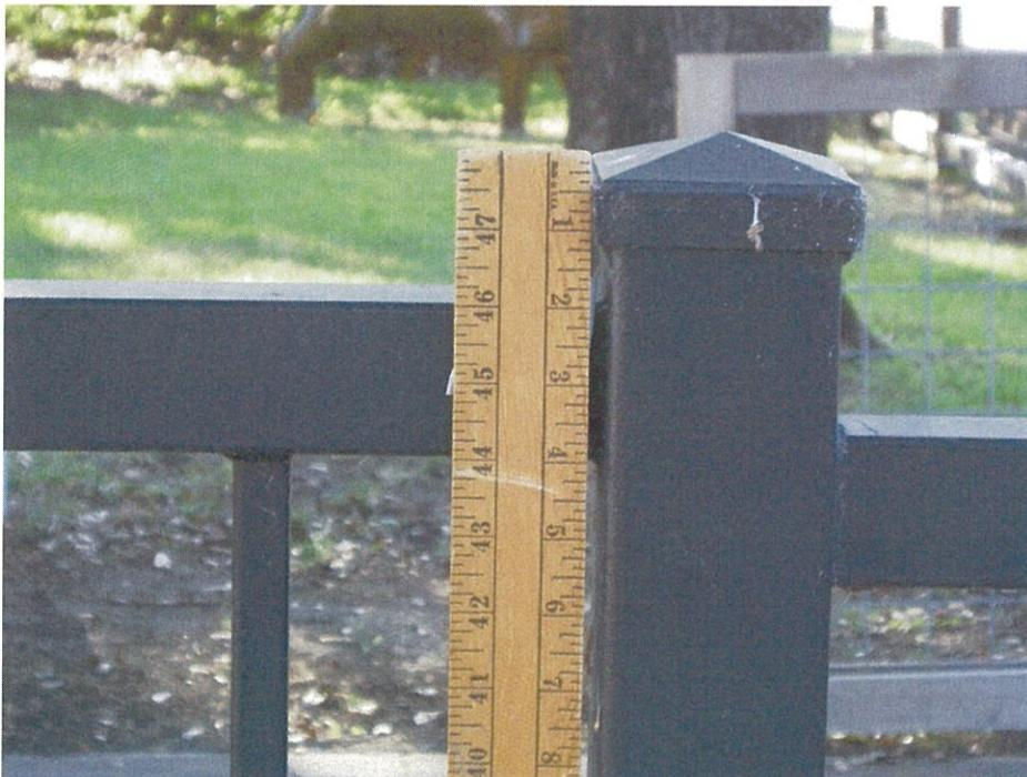
In photo above the height of the Fence Post from bottom fence rail to top of post is 48.5"
