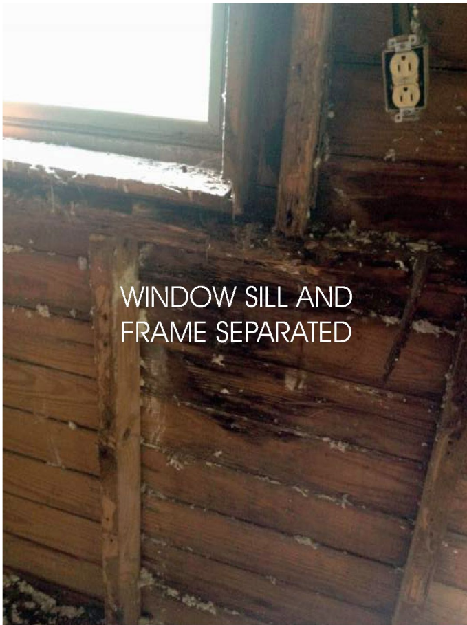
termite and water penetration damage
