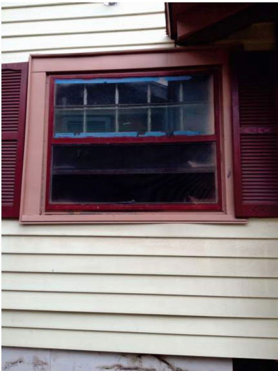
ALUMINUM CLAD AROUND WINDOWS
