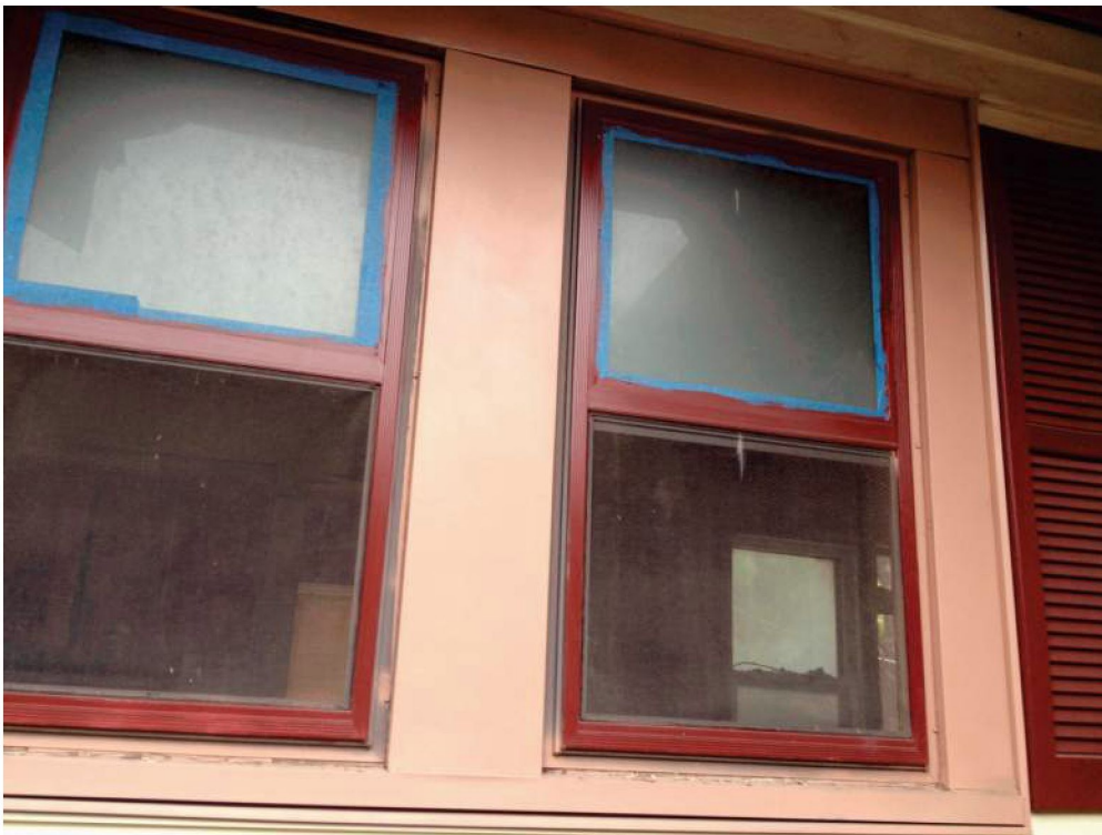
BOTTOM SASHES OF THESE 2 WINDOWS EXPLODED DURING THE FOUNDATION WORK.
