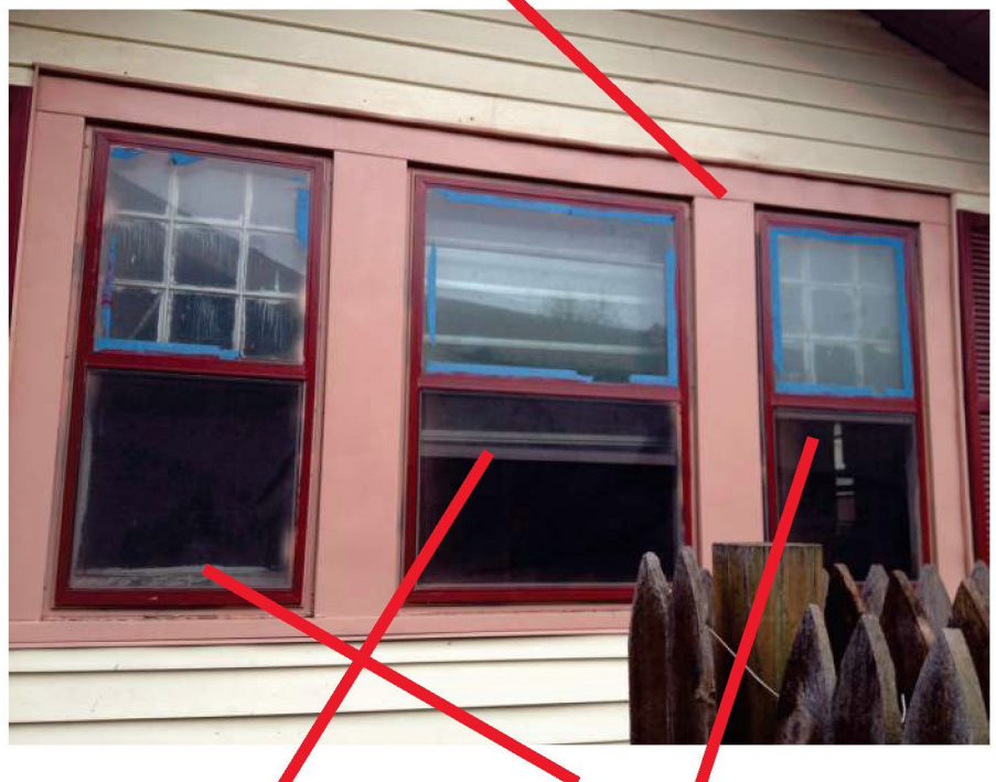
ALUMINUM WINDOW, ROTTEN WOOD WINDOWS
