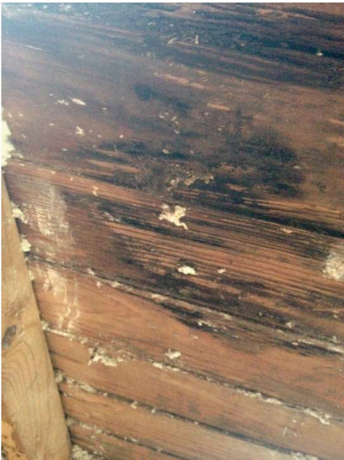
CE167-011(PT) 14 ROTTEN SIDING PICTURED FROM THE INSIDE AFTER SHEET ROCK AND INSULATION REMOVAL
