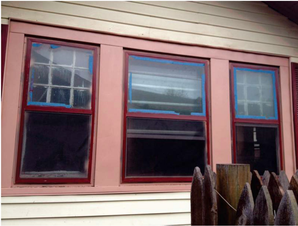
METAL WINDOW IN THE MIDDLE FLANKED BY 2 ROTTEN WOOD WINDOWS
