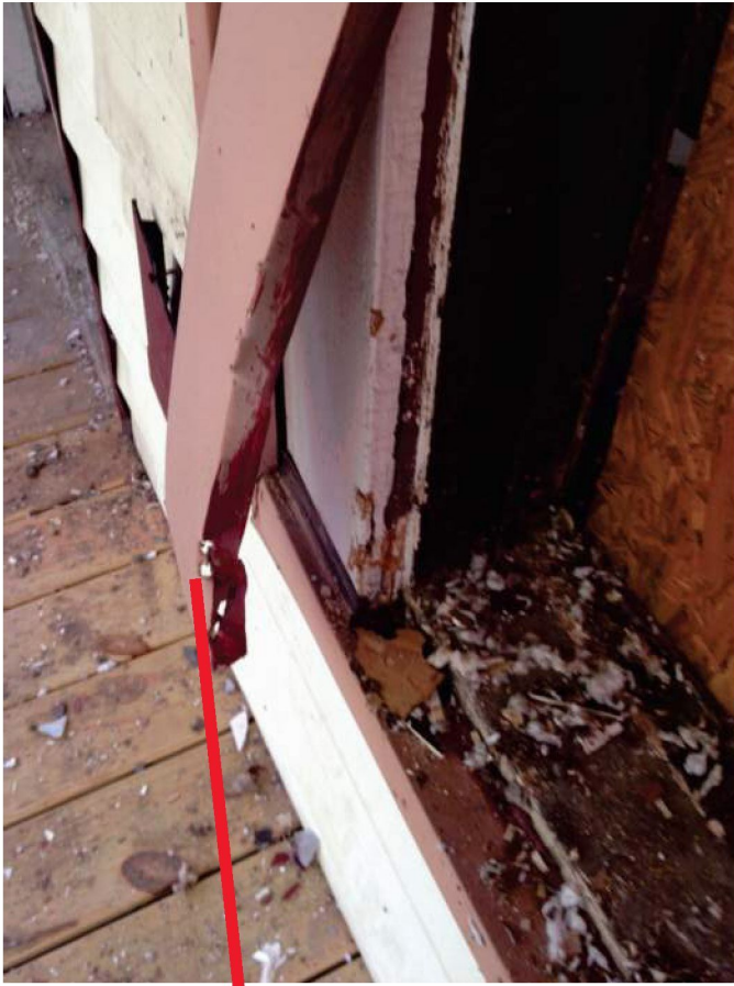
ALUMINUM CLAD AROUND WINDOWS
