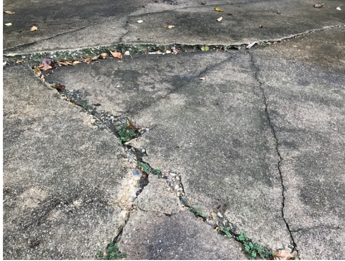
Request #1 – Cracked cement drive, photo submitted by applicant.
