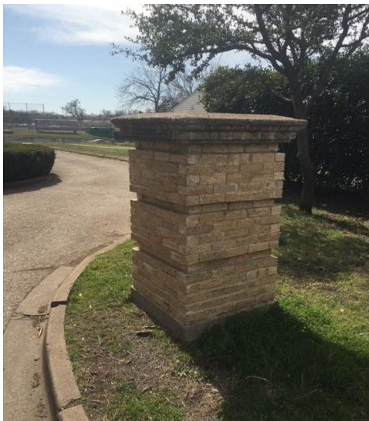
Request #1 – Brick Column Proposed for Relocation (Note the concrete base, which is not present on any other existing brick columns onsite, and which has led the applicant to believe this feature has been moved or reconstructed previously.)
