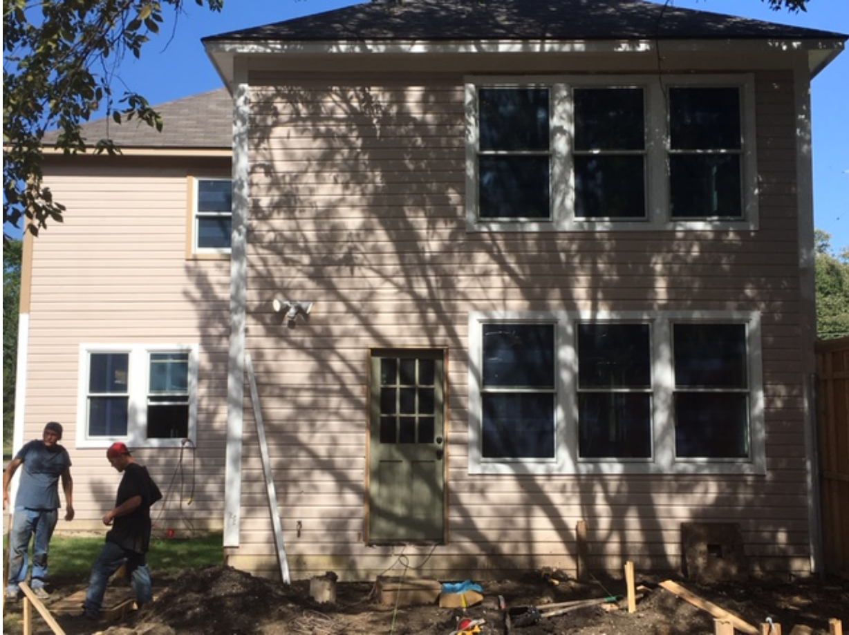
Request #3 – Rear elevation indicated completed siding installation.
