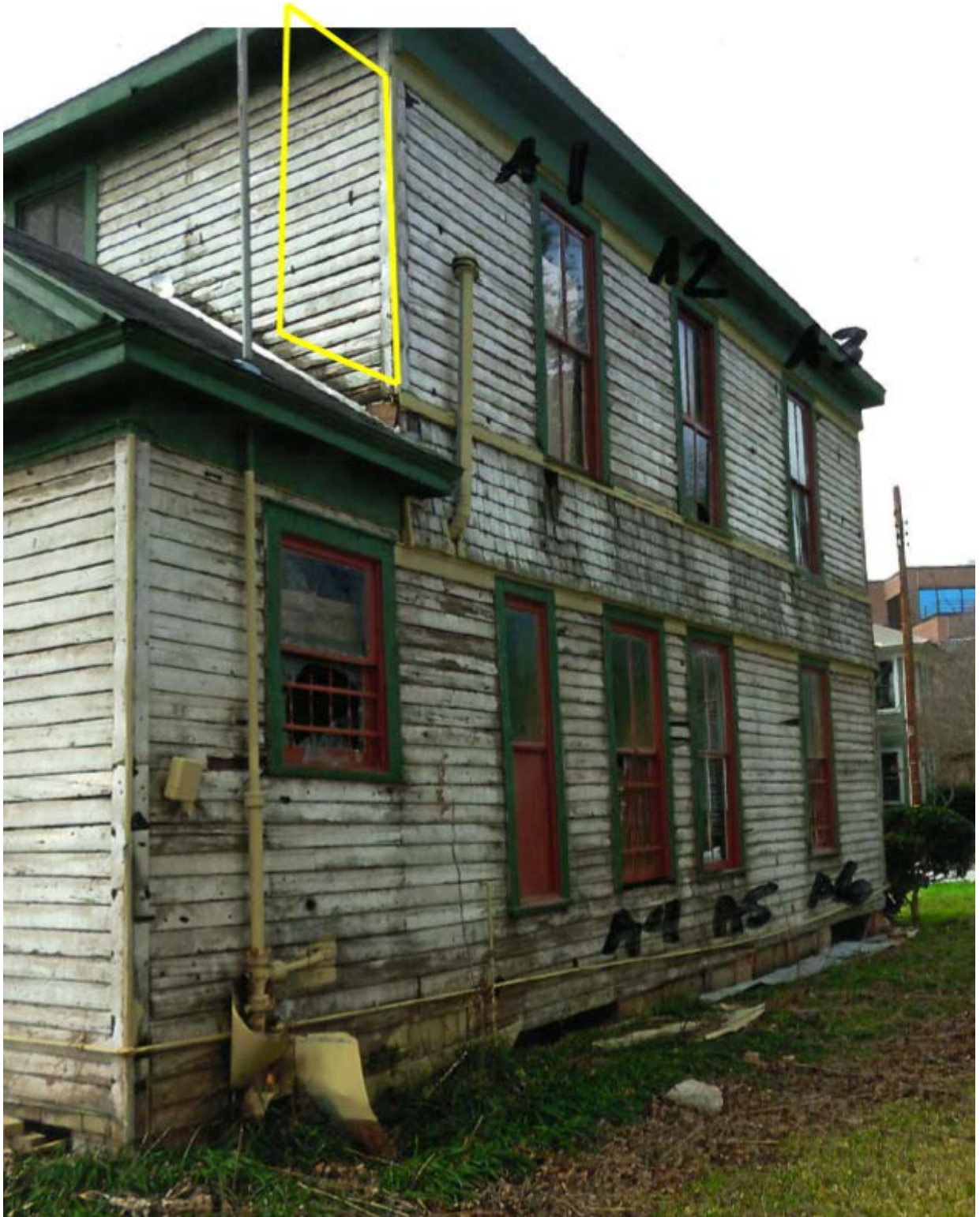
West Elevation Prior to Renovations and Construction of Rear Addition (Approx. location of the proposed window highlighted above in yellow)
