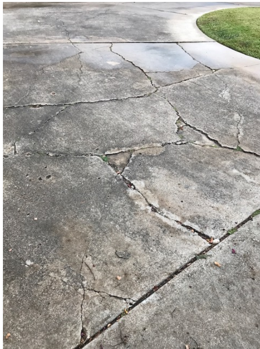
Request #1 – Cracked cement drive, photo submitted by applicant.
