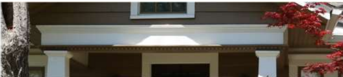
Examples: Minimum 8-inch header beam.
