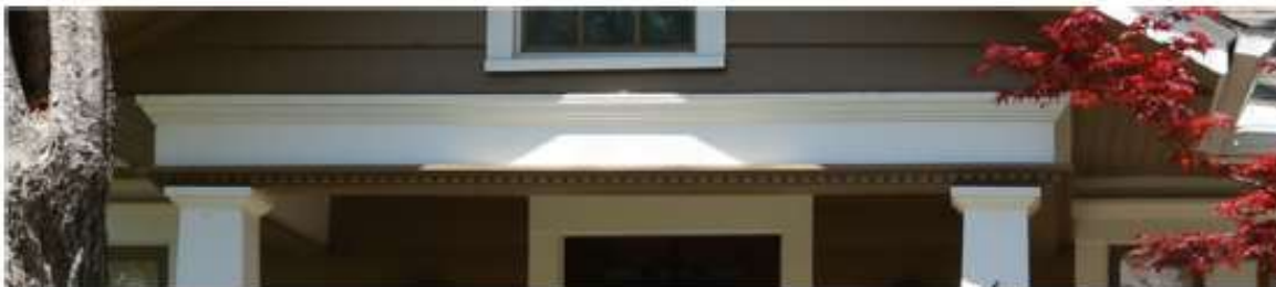
Examples: Minimum 8-inch header beam.
